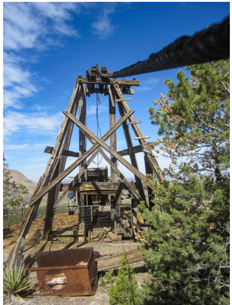
Head Frame and hoist rope at the Nitt Mine (SW)
