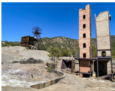
The only parts left of the Kelly Mine – the head frame – ore bin – and smelter (BW)
