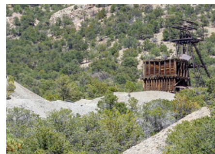
View of the tailings from the Kelly where they mined for Smithsonite (CN)
